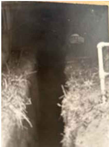
Above: The Shelter dug under our house - June 1967
